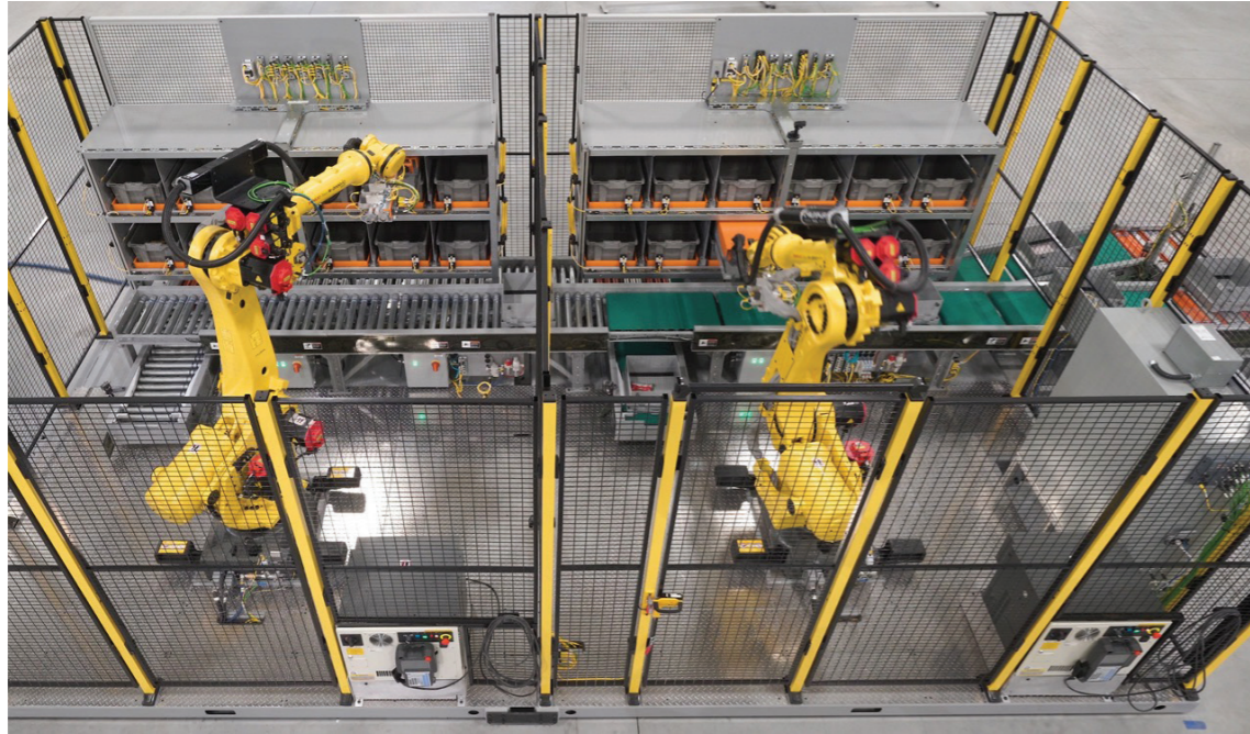
Birds-eye view of a built RFSS in a two-robot configuration. Source: JR Automation
